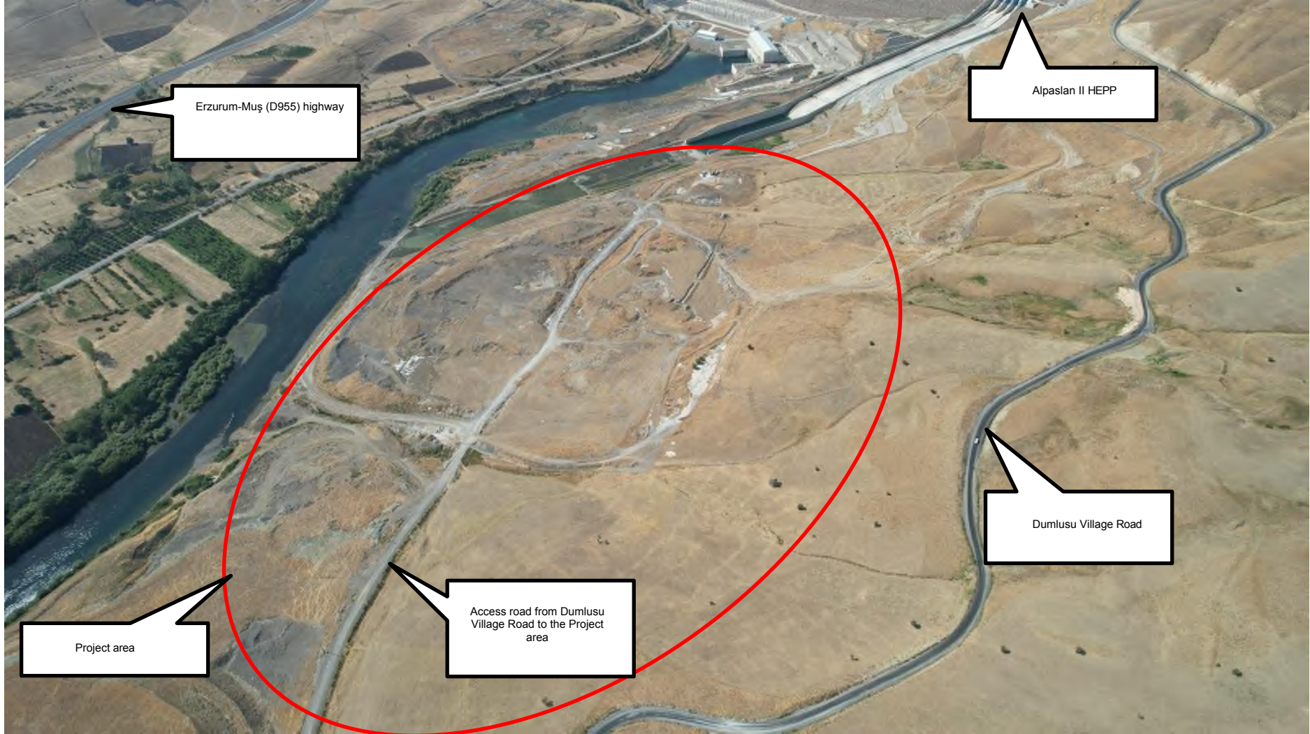
Figure III.1.3.7. View of Existing Roads to be Used within the Scope of the Project-V
