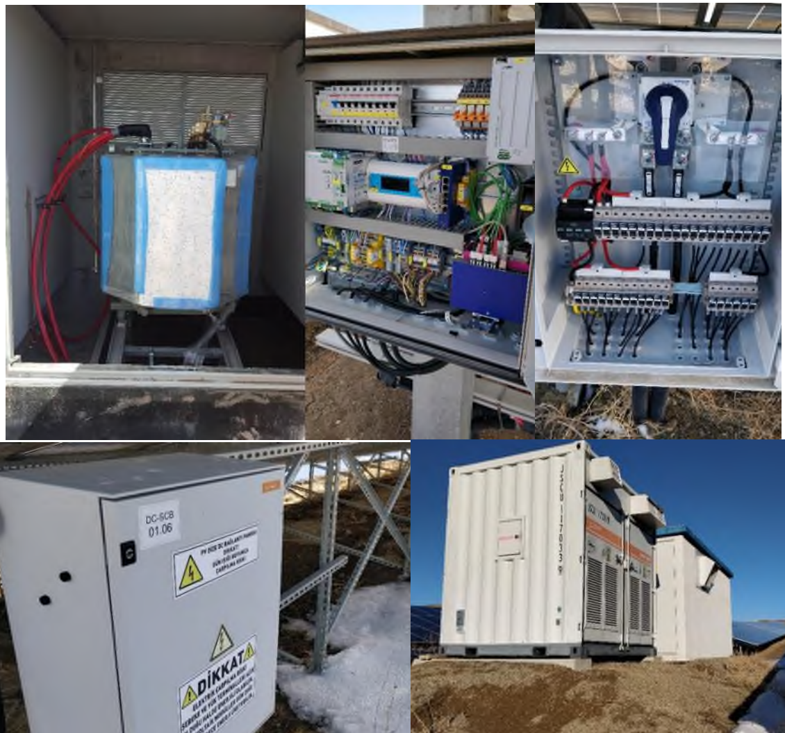
Figure III.1.7.5 Installation of Electrical Connection Equipment Representative Photograph
