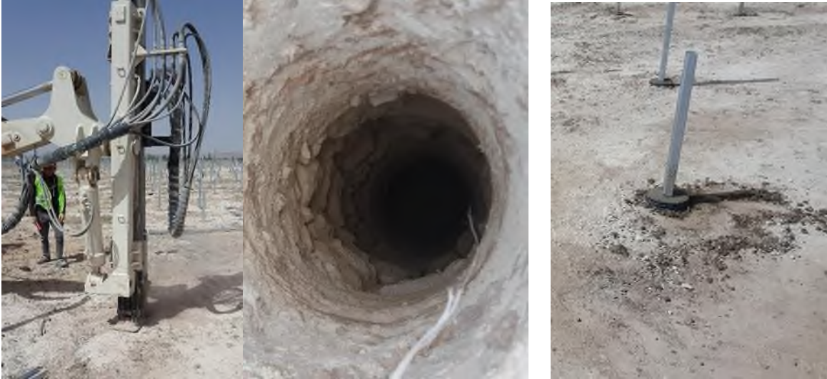
Figure III.1.7.2 Representative Photograph of the Placement of the Carrier System
