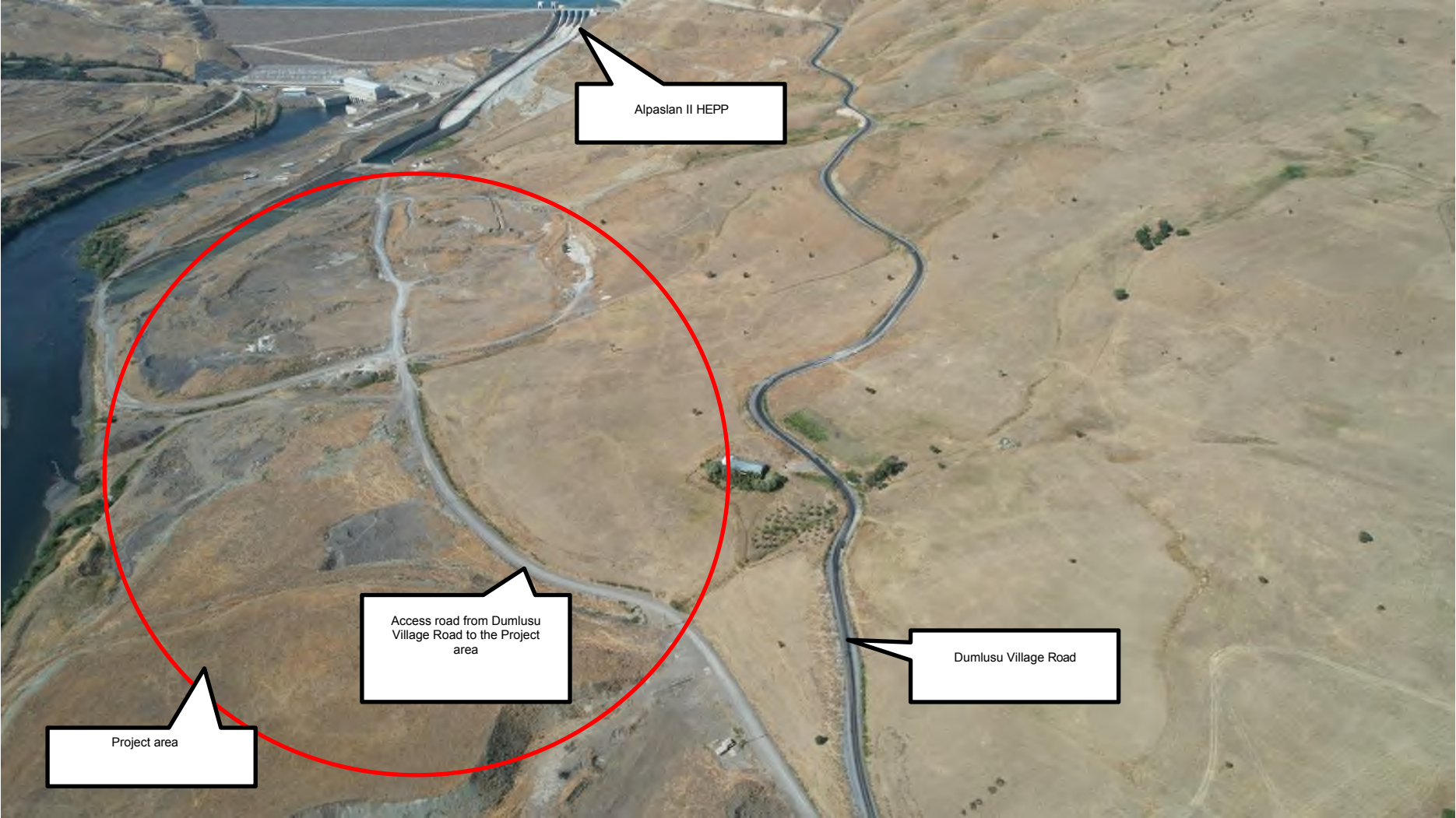
Figure III.1.3.8. View of Existing Roads to be used within the Scope of the Project-VI
