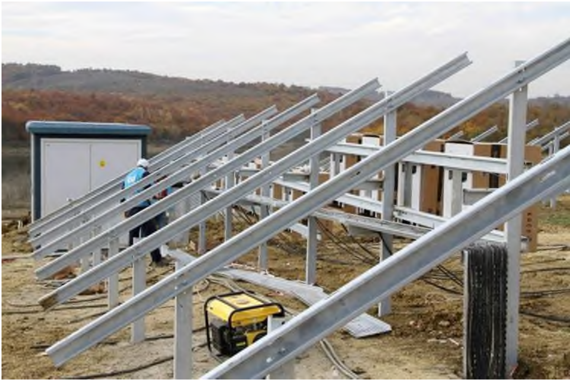
Figure III.1.7.3 Representative Photograph of Carrier System Top Assembly
