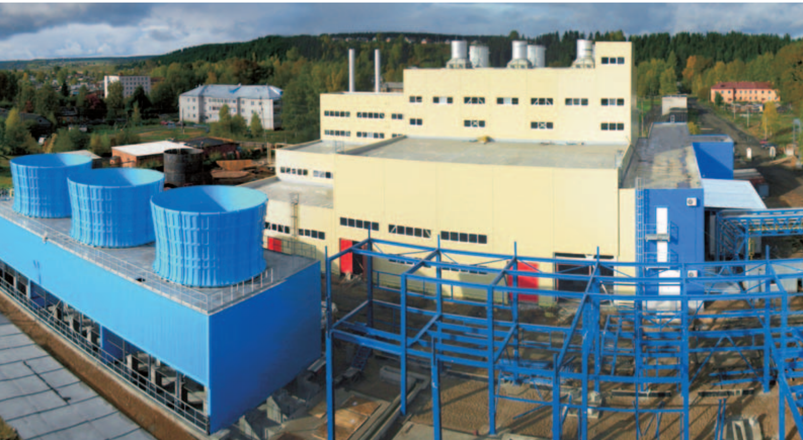
| Construction of the Krasavino power plant, Russian Federation. Supplier: PSG-International, a.s.
