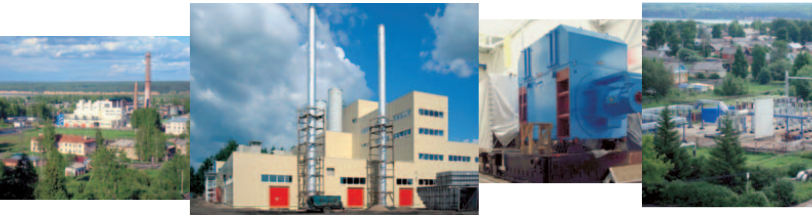
| Construction of the Krasavino power plant, Russian Federation. Supplier: PSG-International, a.s.
